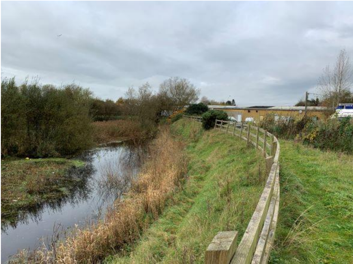
Plate F: Flood defense berm constructed in 2013 on southern boundary of the area infilled as part of the drainage scheme adjacent to the Fort Fergus Stream.
